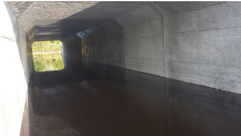
View from inside the aquatic underpass
