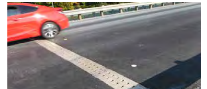
Thanks to this crossing with slots letting the light in, turtles can safely cross the road
